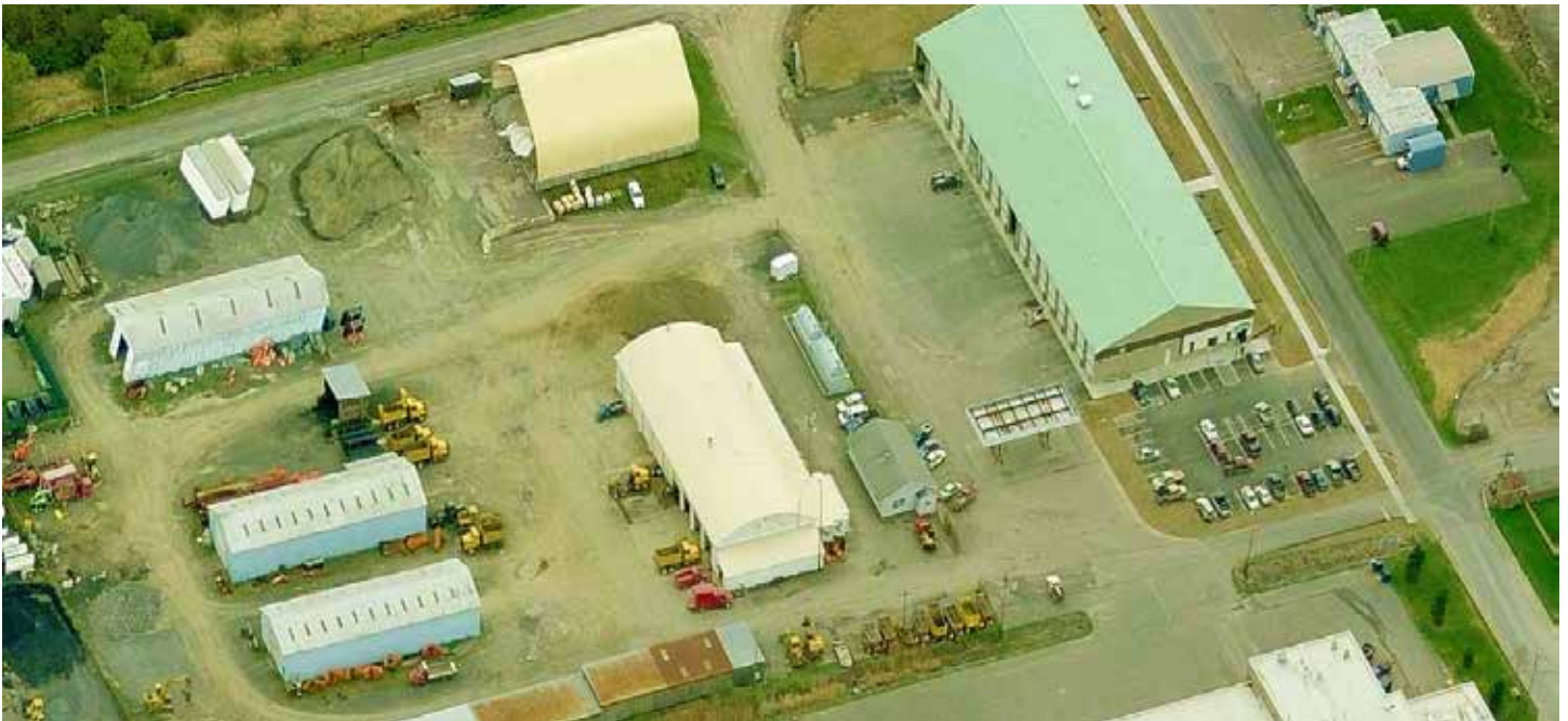
Schuyler County Shared Services Building. This complex includes the Schuyler County Highway Department, Village of Watkins Glen Public Works, Shared Fuel Facility, and Central Garage.
